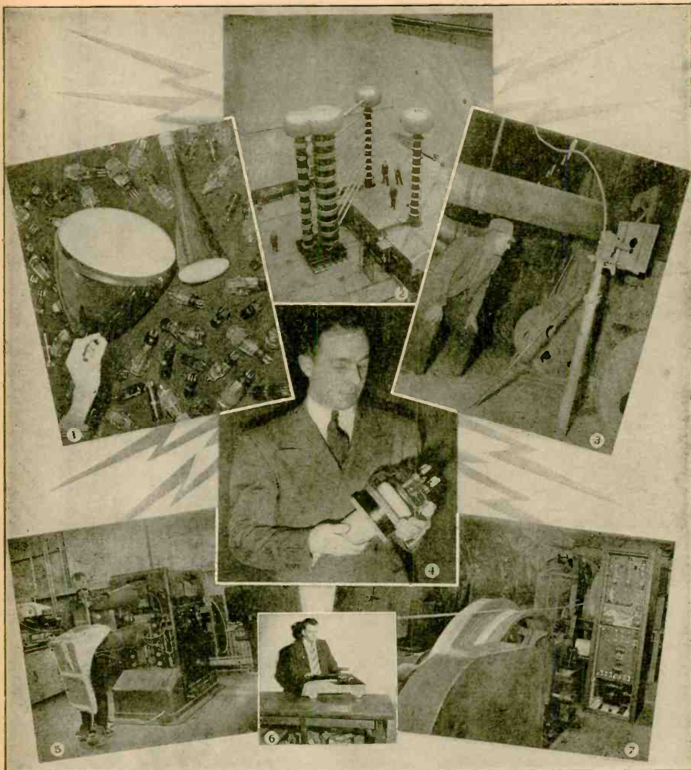
(1) Electronic tubes of various sizes and types as used in television and transmitting. (2) The most powerful X-ray machine in the world at the National Bureau of Standards, has 1.4 megavolt capacity. (3) Phototube system installed in cement kiln for temperature detection and control. (4) Water-cooled tube used in television transmitter. (5) Thyatron control panel controlling spot welder. (6) Herbert Duval, G. E. engineer, with model of new circular-type antenna for portable use. (7) Thyatron motor control alongside cable-stranding machine. These are only a few of the myriads of applications of electronic tubes and devices in modern industry. The art is growing by leaps and bounds and will open up unknown worlds for man's inventive genius.
